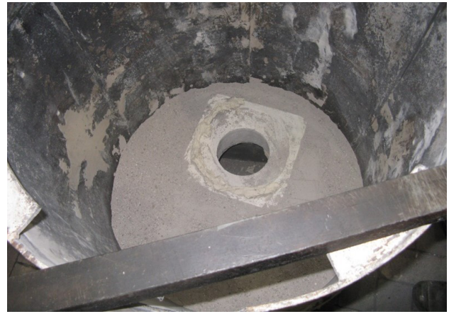
Figure 1. Wellblock L0 installed in the ladle bottom
