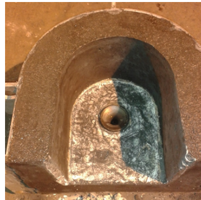
Figure 9. Conventional Nozzle in a runner of an Autopour Furnace, installed from the top
