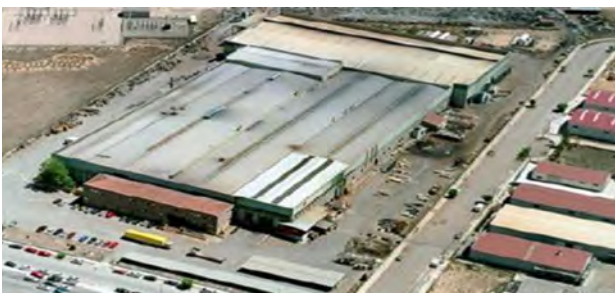
Figure 1. PYRSA Monreal del Campo facility, Teruel, Spain.
